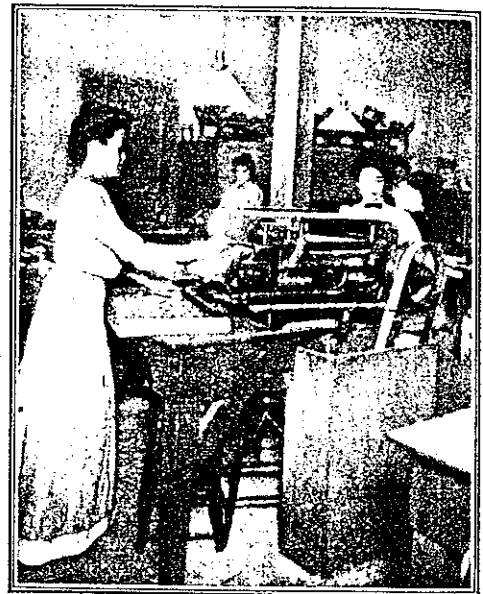
In the "noodle" machine the lumps of "dough" are whirled between two belts and come out in small pipes.
